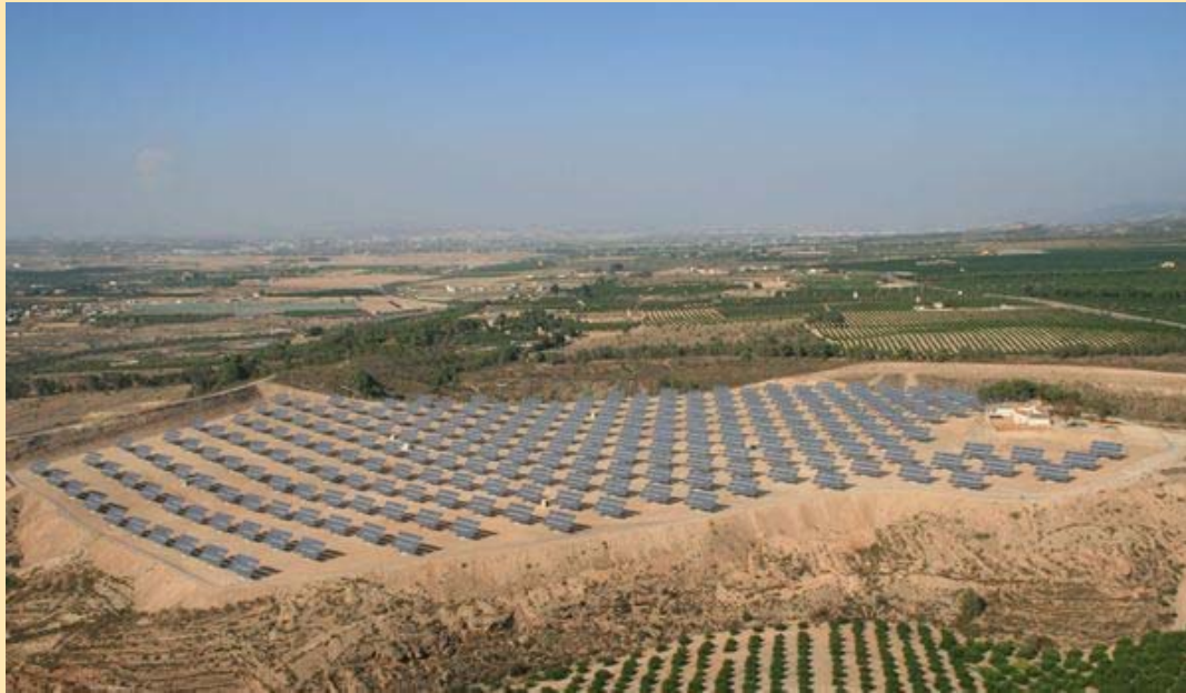
El Cañarico Plant
